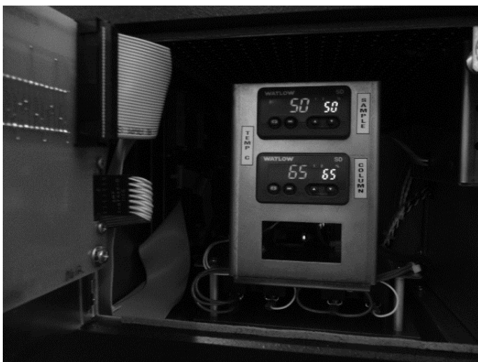
Figure 2-3: Internal Temperature Controllers
